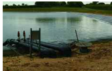
The new reservoir supplies irrigation to the estate’s root and vegetable crops and is part of a long-term view of farming taken by the MacNicol family.
